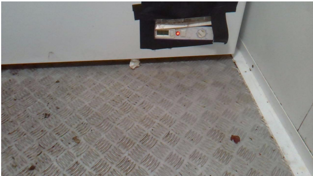
Loose tape to control panel to chest freezer
