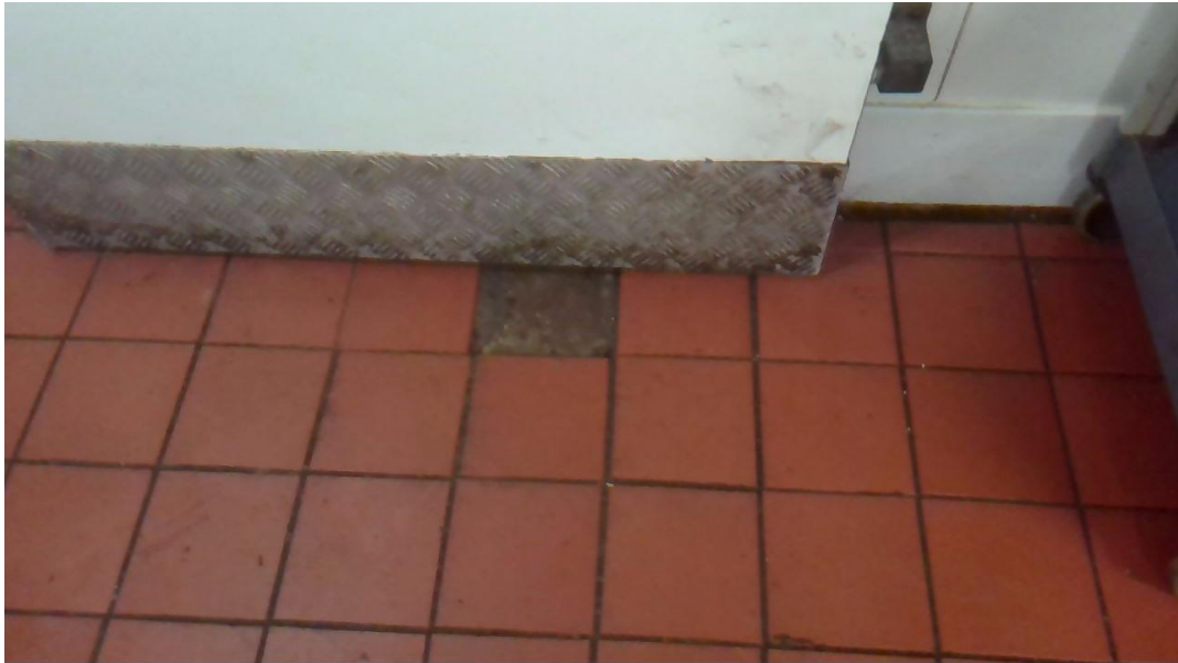
Missing tile to floor
